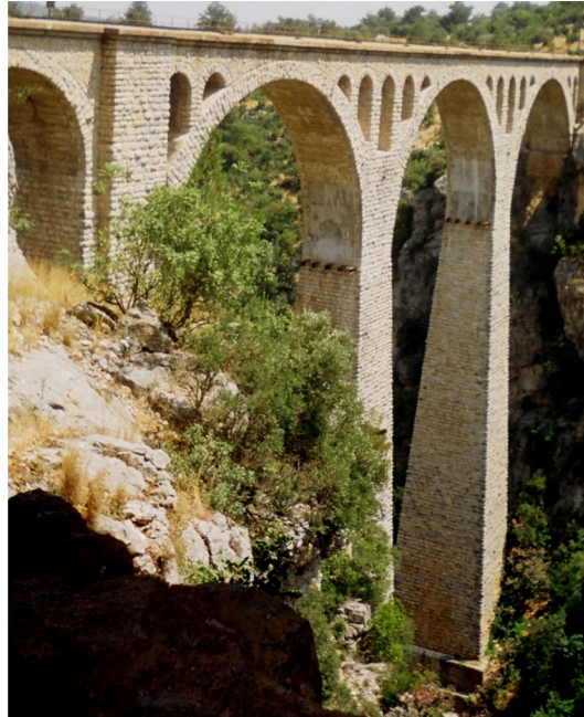
Fig. 2 Detail view of spans of 36 m
