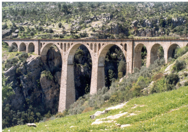
Fig. 1 General view of the Hacikiri bridge
